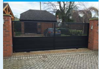
GARITA - SLIDING GATE
