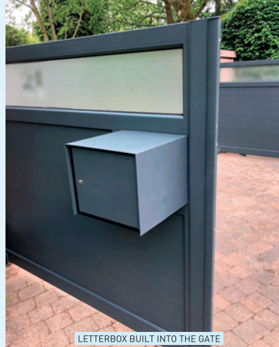
LETTERBOX BUILT INTO THE GATE
