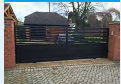
GARITA - SLIDING GATE
